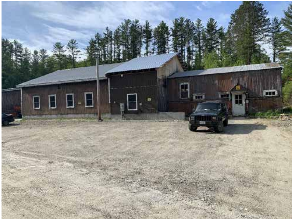
Main Entrance exterior
