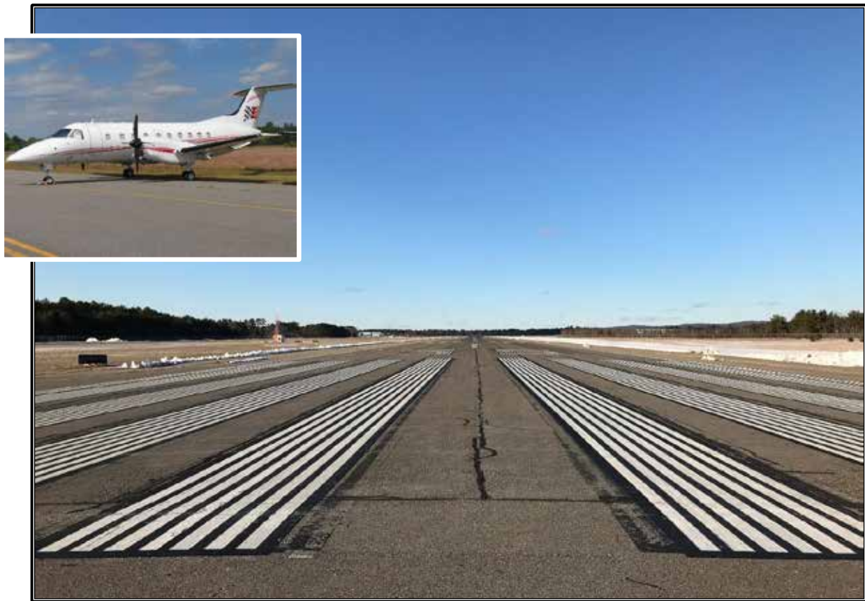
Figure 3: View of Concord Municipal Airport's Runway 17-35.
