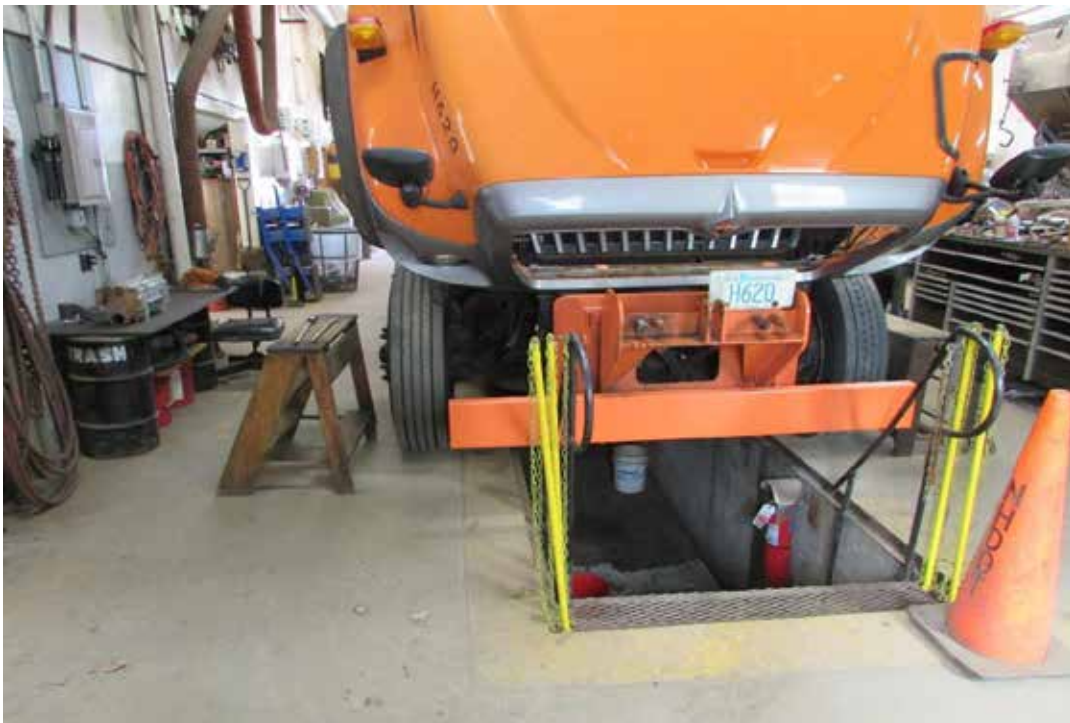
Lancaster – Low ceilings so employees work in a “pit”. The ceilings are too low to raise the dump body of have use for mobile lifts that would improve ergonomics.
