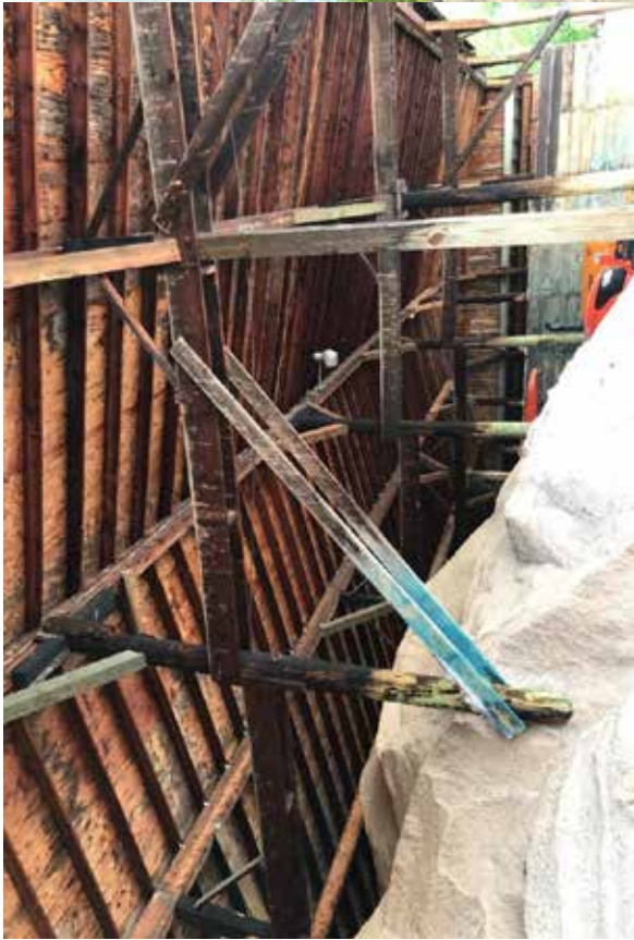
North Hampton (612) – Internal structure
