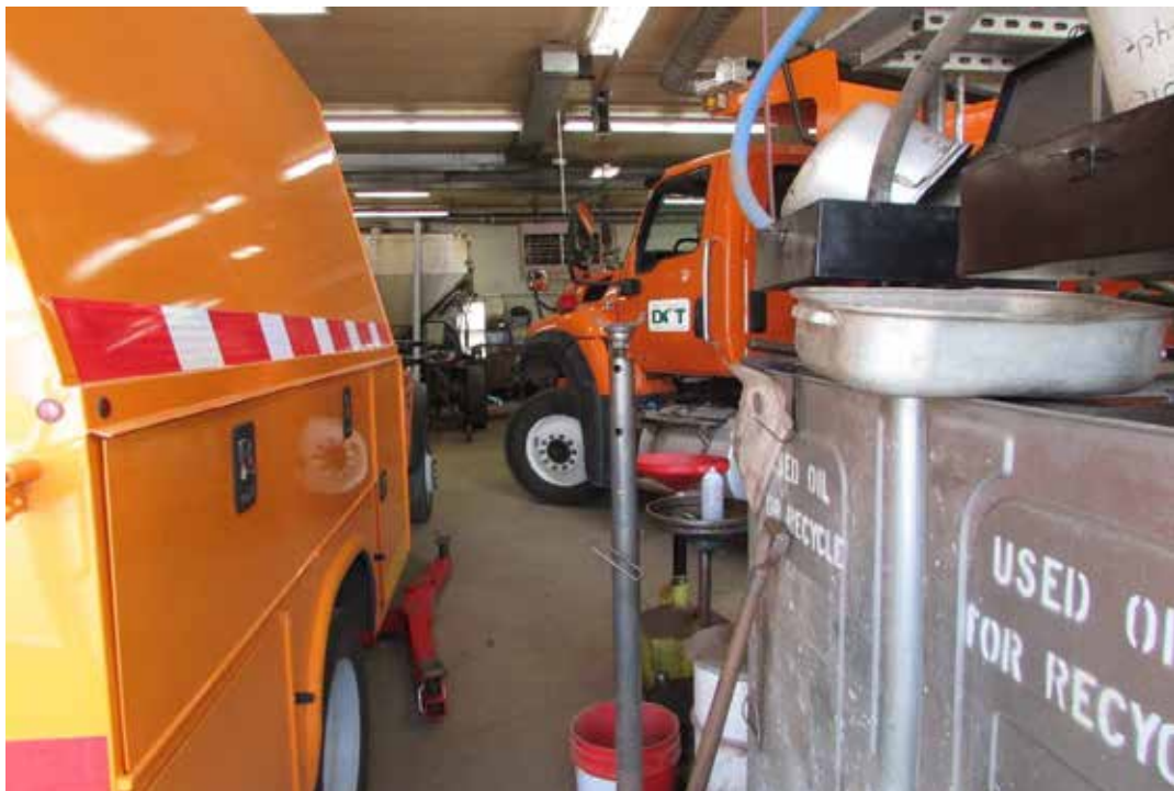
Lancaster – Lack of room to work safely
